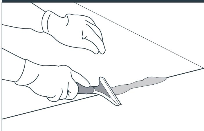
After any construction work has been completed the floor should be cleaned. The expanded foam should only be removed with a scraper when the building is weathertight to prevent water ingress and edge swell.
