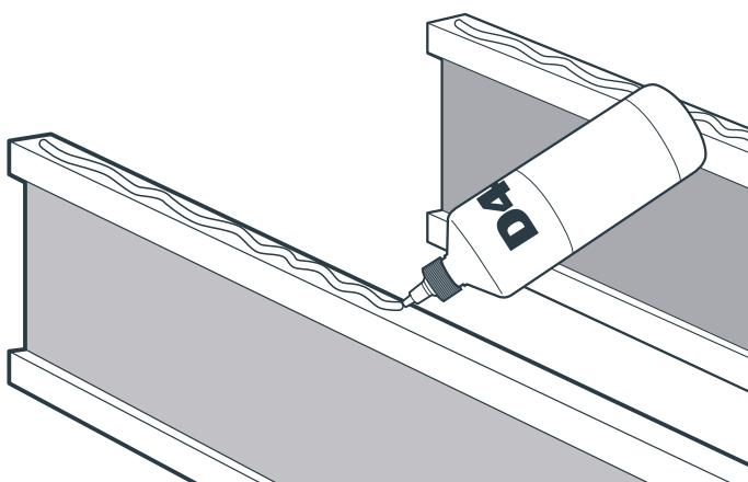
Apply one continuous bead of D4 rated (EN 204) foaming adhesive to the top of the joists and noggins corresponding to the area of the 1st panel to be installed.
